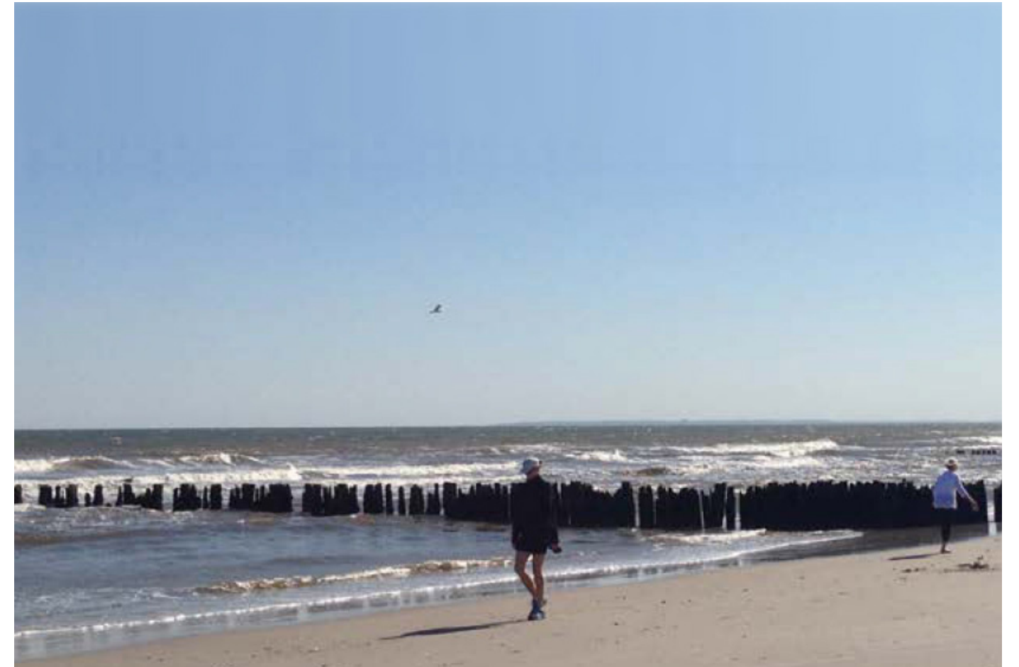
GROINS ALONG THE ROCKAWAY PENINSULA SOURCE: NYC DCP, 2013
